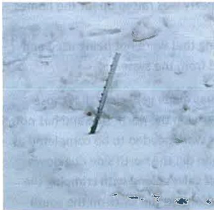
curb stop not in use
