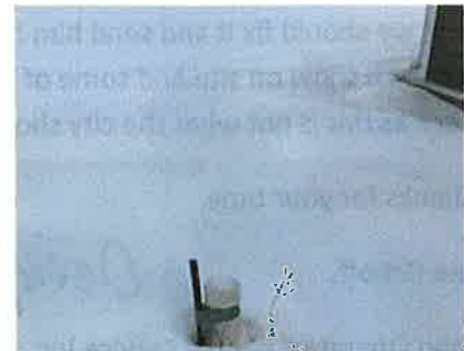
Sewer and water line not in use
