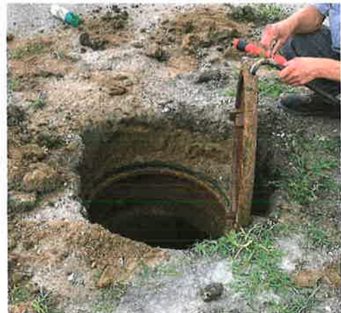
buried manhole structure
