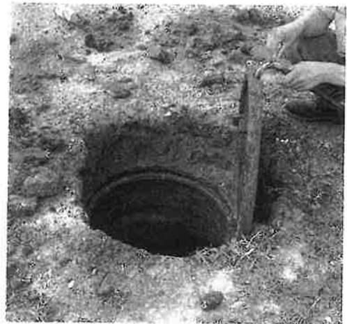
buried manhole structure
