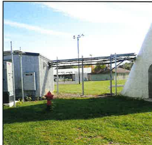
5 CABLE BRIDGE PHOTO
