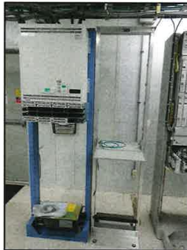
5 POWER PLANT PHOTO
