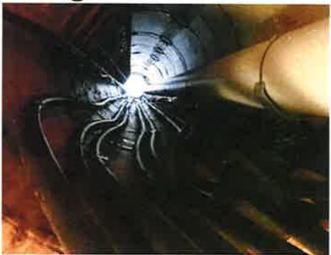
4 DRYWELL TUBE PHOTO
