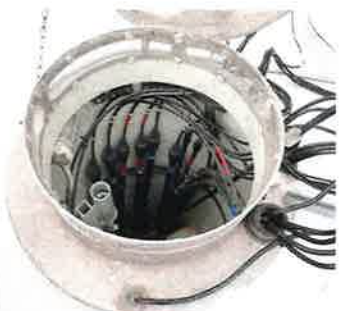
6 DRYWELL HATCH PHOTO
