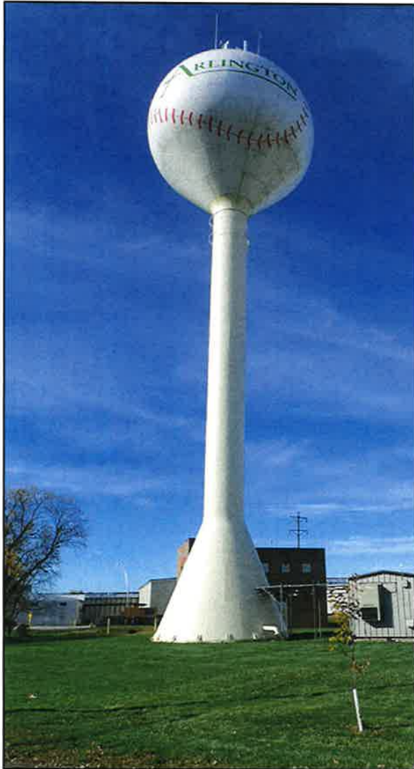
1 OVERALL TOWER PHOTO
